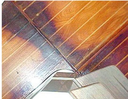
Any bleaching must be done after initial sanding, but before final sanding and detailing is complete. It will require time for the wood to dry before moving on.
